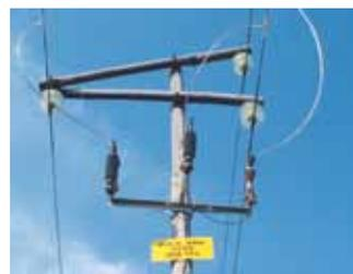
Figure 16: The installation of drop-out line surge arresters.
