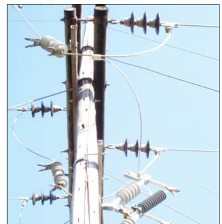
Fig. 2: Surge arrestors provide high reliability protection for overhead lines.
